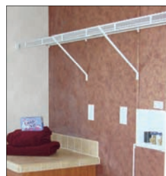
WIRE SHELF AT WASHER/DRYER AREA
