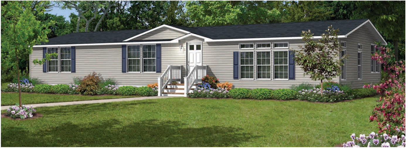
LARGE EYEBROW DORMER, WHITE TRIM, TRANSOME WINDOWS ON A STEP-DOWN
